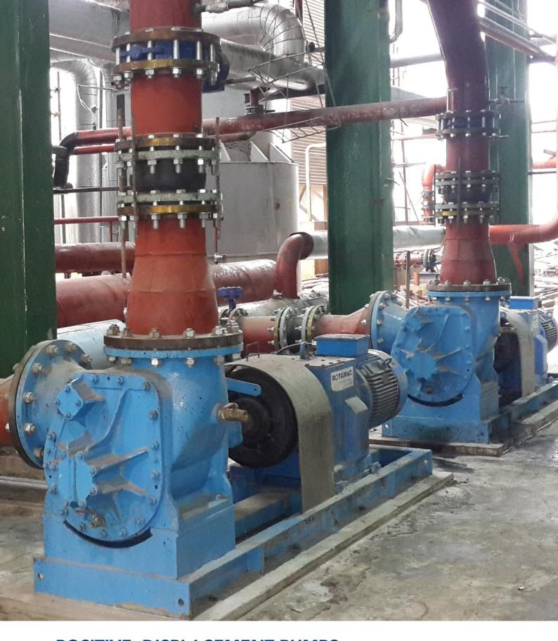
POSITIVE DISPLACEMENT PUMPS FOR HIGH VISCOSITY LIQUIDS
