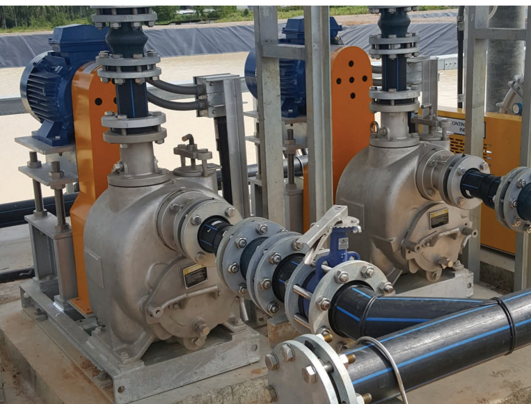
Example of use : Self-priming pump, discharge sizes three inches in stainless steel 304 material for wastewater. Rated point 70 m 3 /h - 20 m - 1800 rpm - 11 kW
